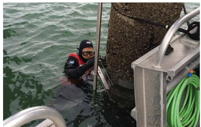
*A diver installing the 400 kHz 2D Profiler clamp onto the piling.*
